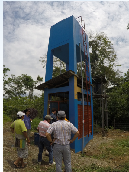
Neighboring community well system.
